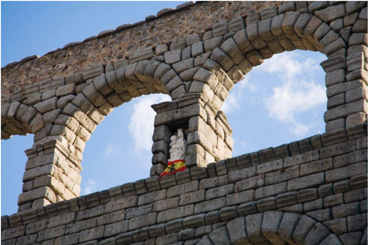
Aqueduct (Acueducto de Segovia). 1st century AD. Sites and Photos. Artstor. https://jstor.org/stable/community.15221758 .
